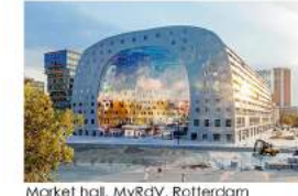
Market hall, MVRDV, Rotterdam
